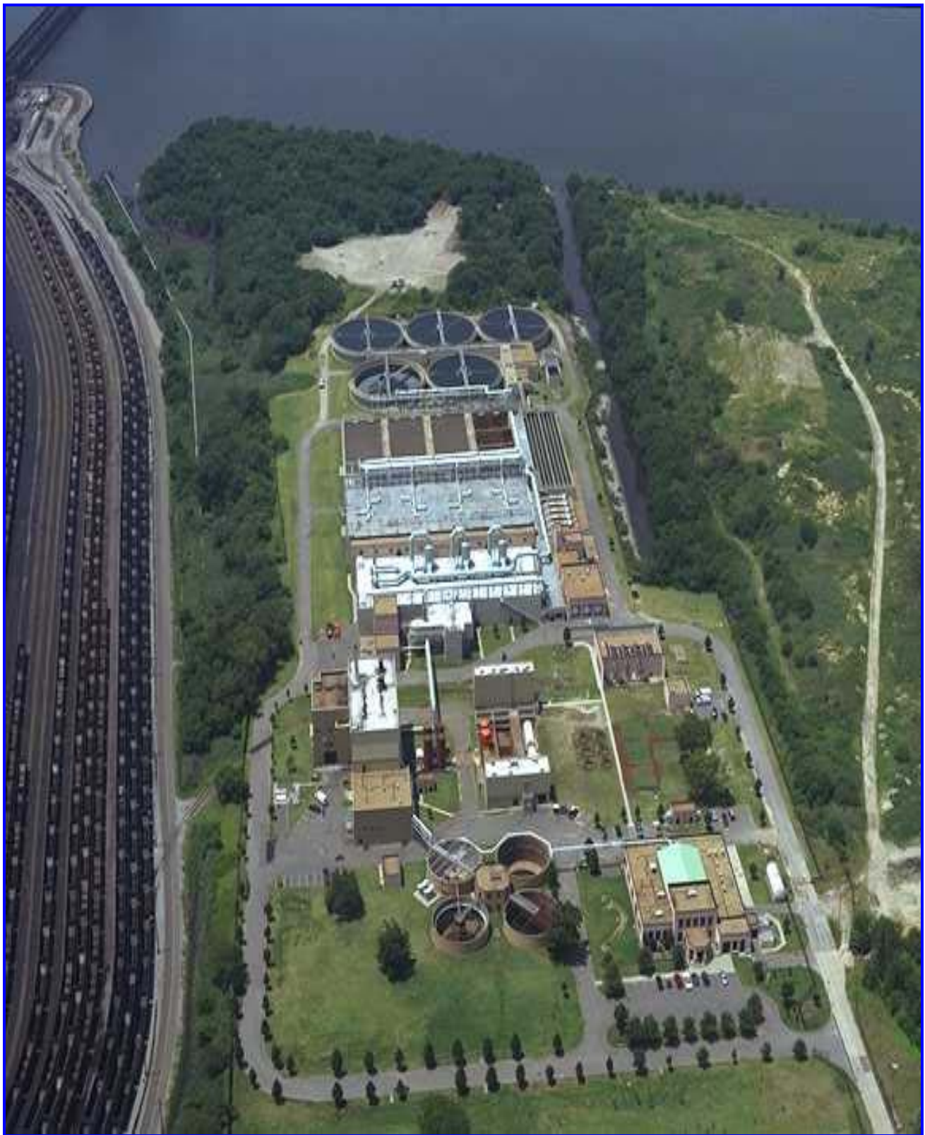
Figure 1: Virginia Initiative Plant (VIP) Aerial Photo
